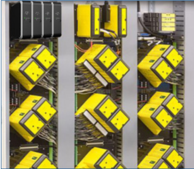
DeltaV SIS logic solvers mounted vertically.
