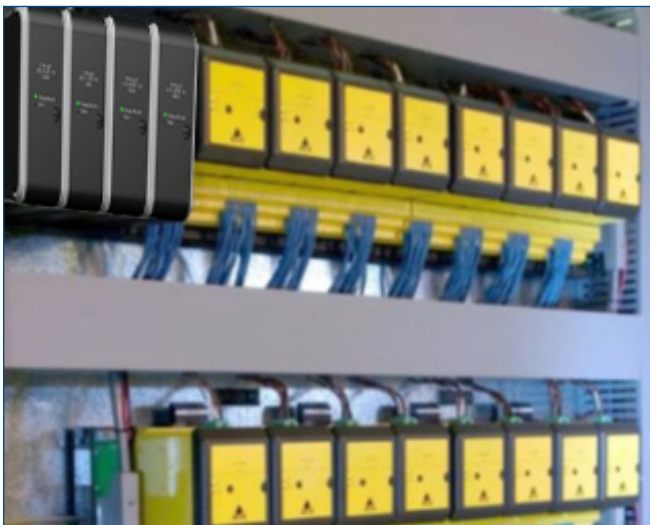
DeltaV SIS logic solvers mounted horizontally.
