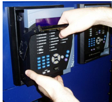
FIGURE 3-7: Slide Unit out of Case
