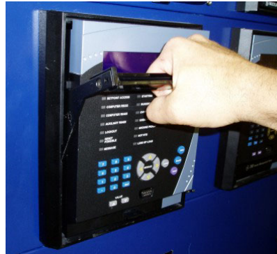
FIGURE 3-6: Rotate Handle to Stop Position
